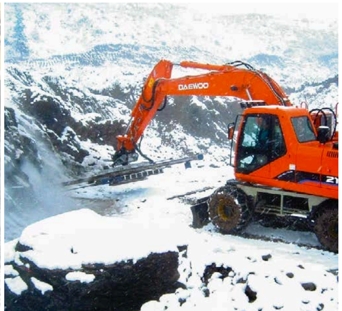
HB5 nailing in the mountains
