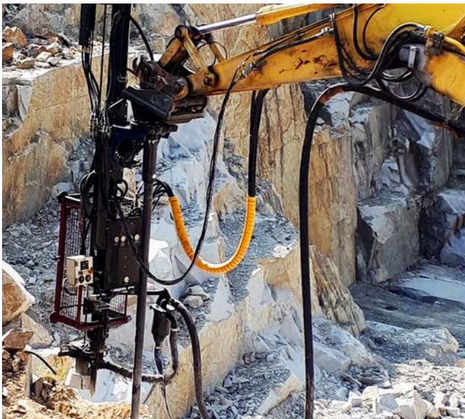
HB5 drilling in a granite quarry
