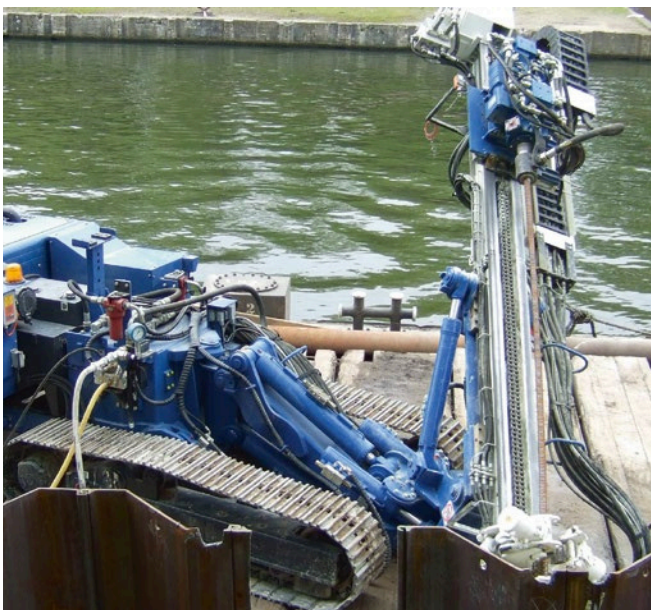
HB20 drilling Ø52 mm (2 inch) threaded hollow bars
