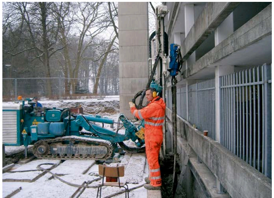
HB15 drilling \varnothing 101 mm (4 inch) casings
