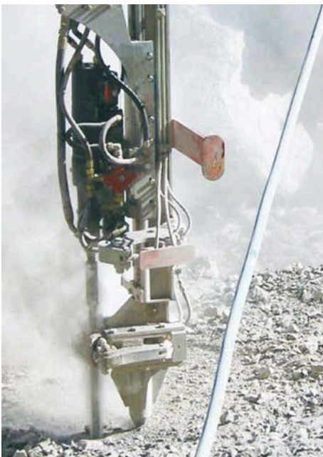
HB15 drilling in a quarry
