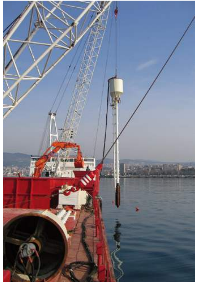
Off shore application: harbour of Trieste Italy. Bottom feed stone columns for sea bed consolidation.
