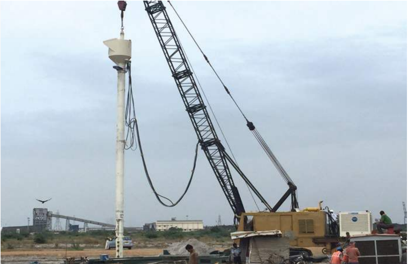
STA Power Pack separated from base machine. Wet Top Feed Mathura India.
