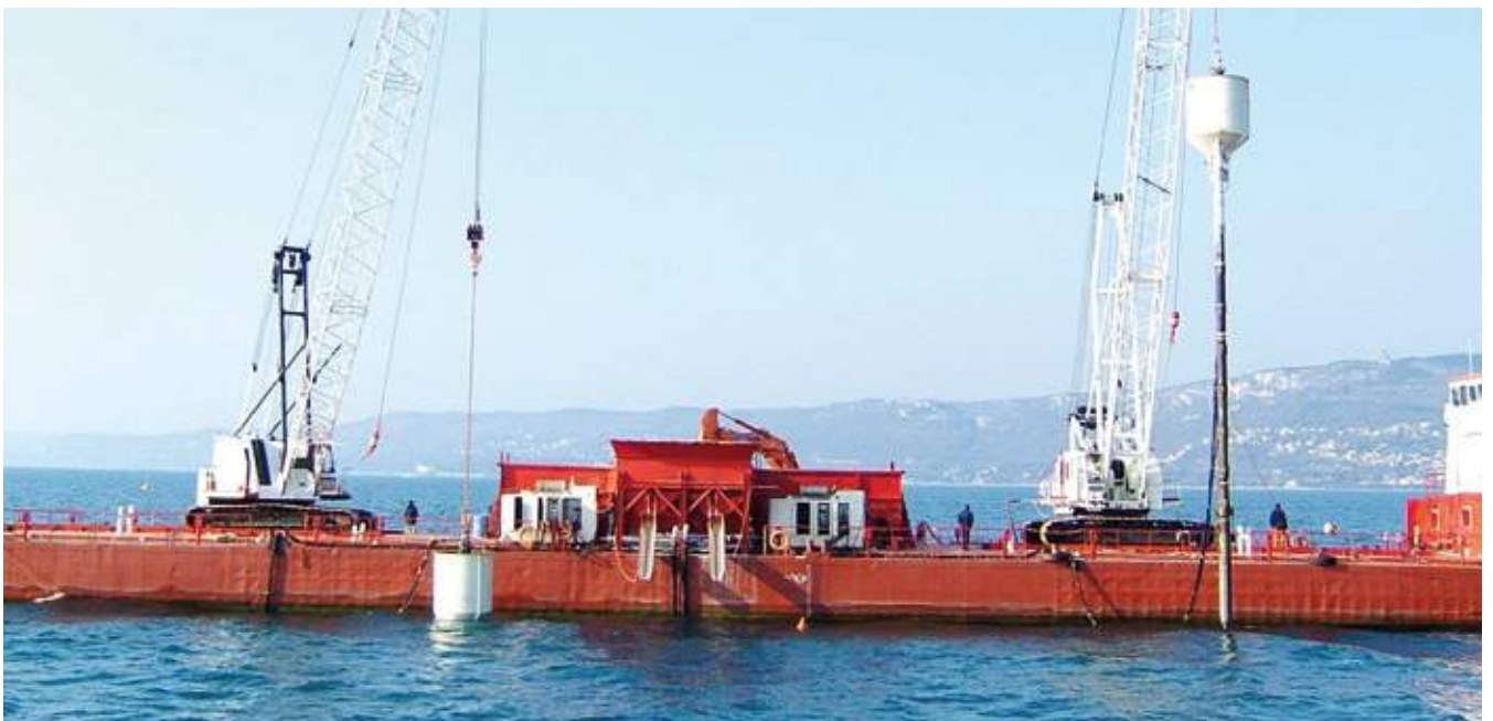
Off shore application: harbour of Trieste Italy. Bottom feed stone columns for sea bed consolidation.
