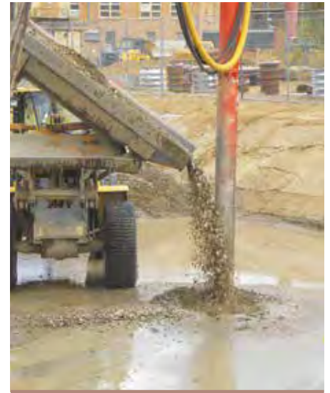
Two Vibrolances VL40S sets for the construction of a new hospital in Quebec, Canada. The project consists of working on the soil treatment by installing 12 000 linear meters of stone columns. Each Vibrolance had a productivity of 150 linear meters a day.
