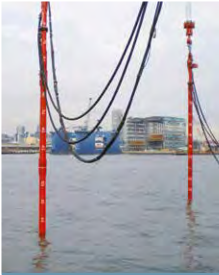
Two Vibrolances working in the compaction of 17 million m 3 reclamation sand at an underwater depth of 15 to 20 m. The soil improvement treatment is required for building a new 6 km long quay, Singapore .
